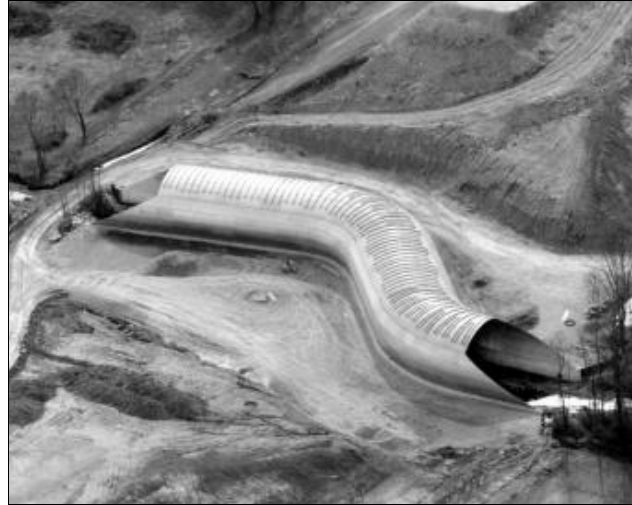
Figure 5.3. Culvert with a horizontal bend (Contech).
