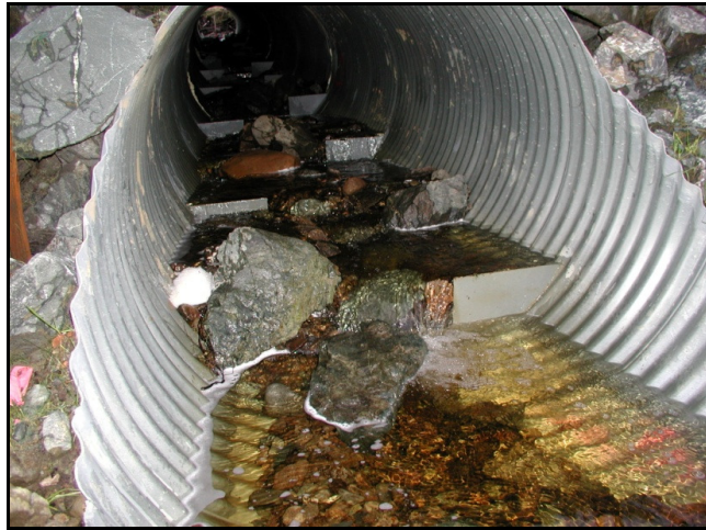
Figure 5.6. Alternating baffles.
