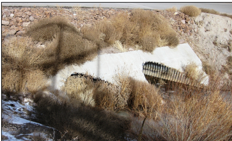
Figure 5.20. Slope paving around a mitered inlet.
