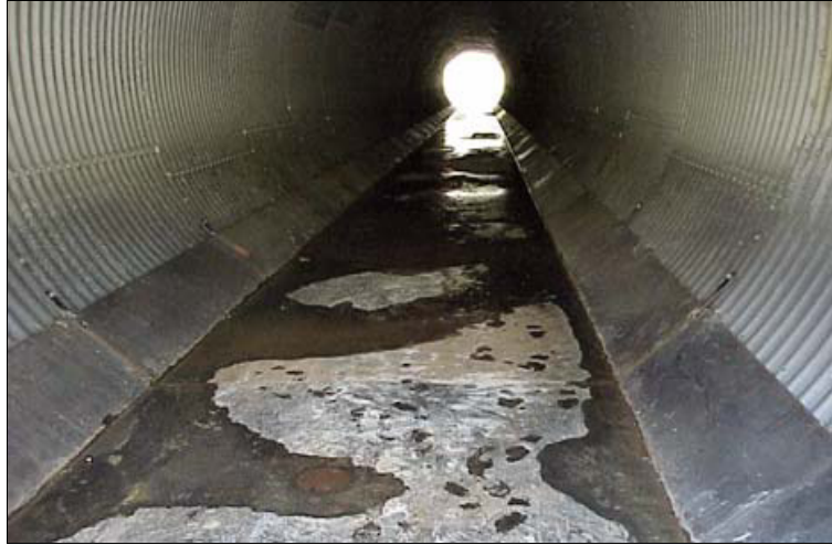
Figure 6.18. Invert repair of CMP using steel plating.
