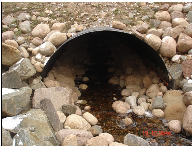
Figure 1.13. Embedded culvert (from WI DOT)
