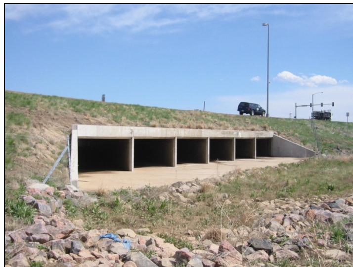
Figure 5.17. Multiple barrel box culvert.
