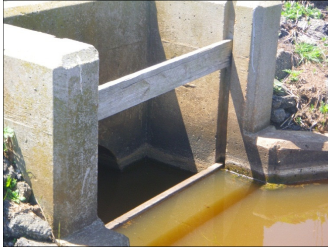
Figure 5.1. Culvert as outflow control device.
