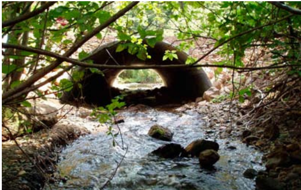
Figure 4.4. Completed open-bottom installation (from USFS 2008).
