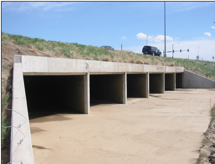
Figure 1.22. Multi-cell box culvert.
