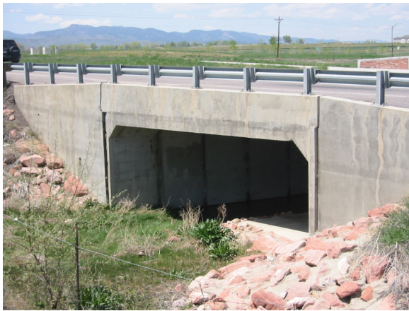
Figure 1.6. Concrete box culvert.
