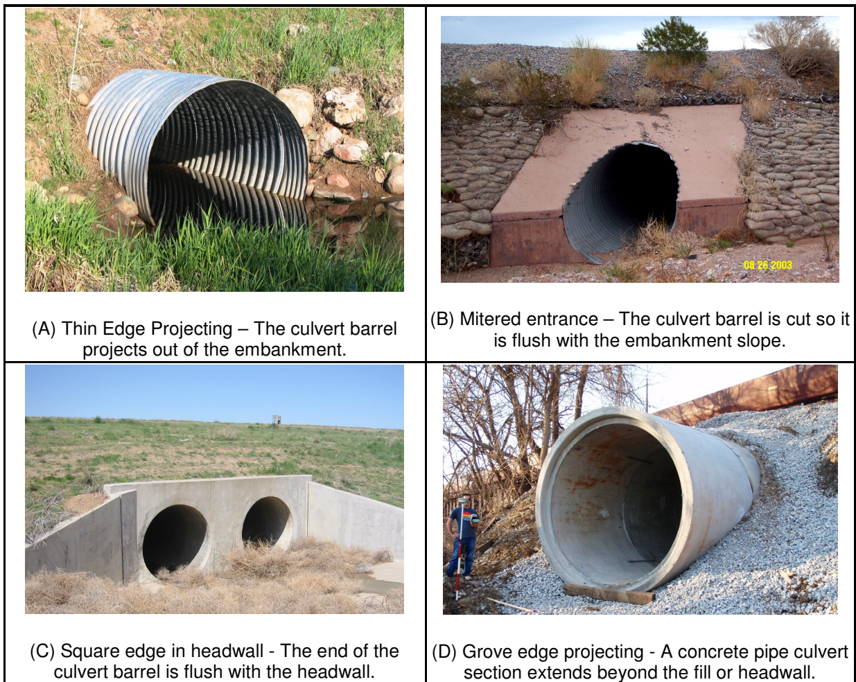
Figure 3.2. Typical inlet configurations.
