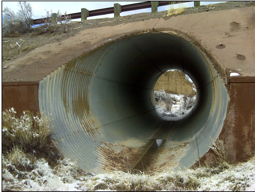
Figure 1.21. Structural plate culvert.
