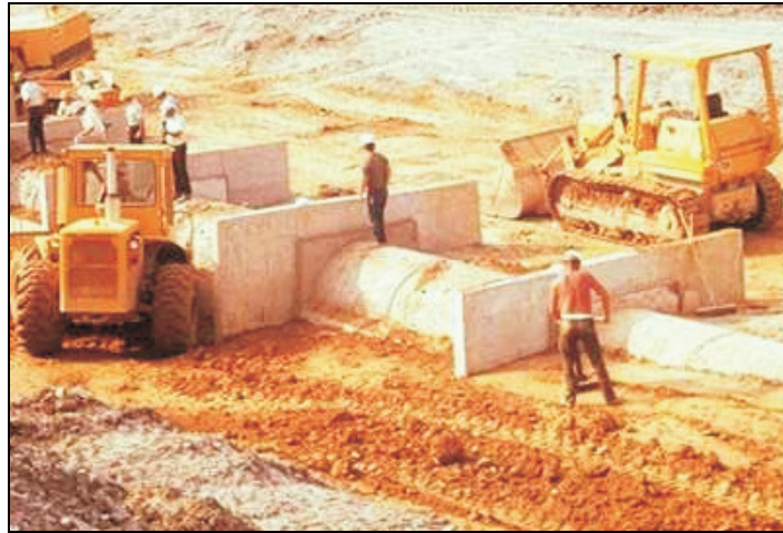
Figure 5.21. Anti-seep collars (FEMA 2005).
