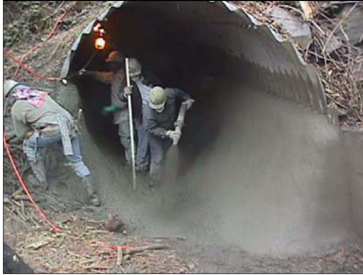
Figure 6.16. Spray-on mortar liner installation via person-entry (from CALTRANS).
