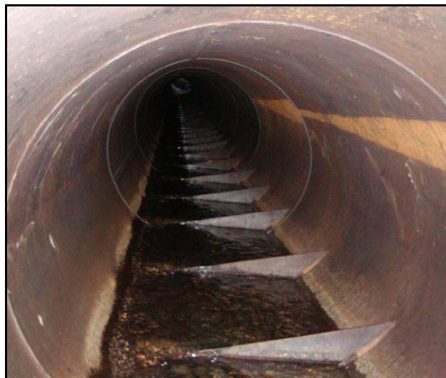
Figure 5.7. Angled baffles (from FishXing Users Manual)
