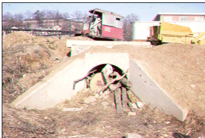
Figure 6.3. Severe debris blockage.
