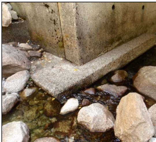
Figure 6.9. Exposed spread footing in an open-bottom culvert.
