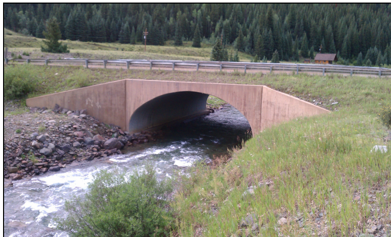
Figure 1.12. Open-bottom culvert.
