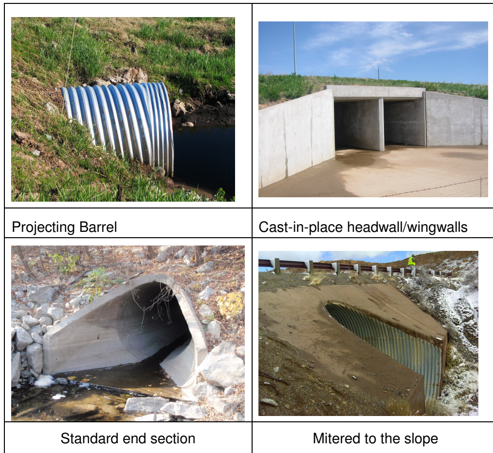
Figure 1.8. Four standard inlet types.
