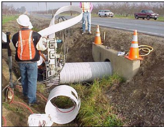
Figure 6.11. Example of a spiral wound liner installation with restricted access at culvert end.
