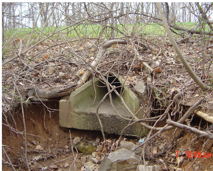
Figure 6.8. Scour hole at outlet of an RCP culvert.
