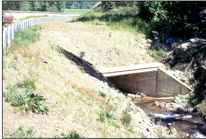
Figure 5.16. Fill warped to avoid inlet skew.
