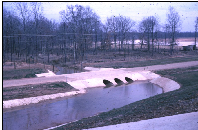
Figure 1.15. Vented low-water crossing.
