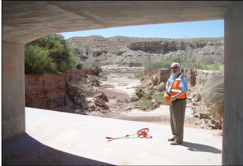
Figure 5.11. Stream degradation downstream of culvert outlet (from Utah DOT).
