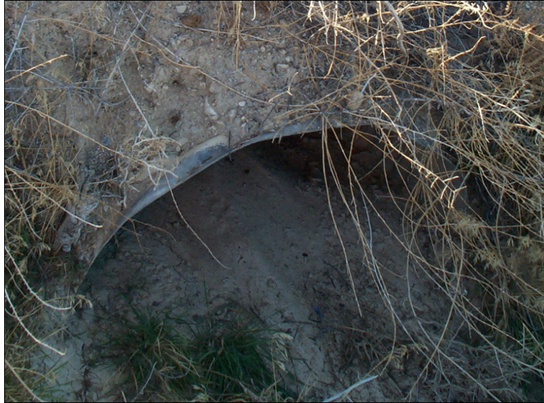
Figure 5.12. Excessive sediment deposition in culvert.
