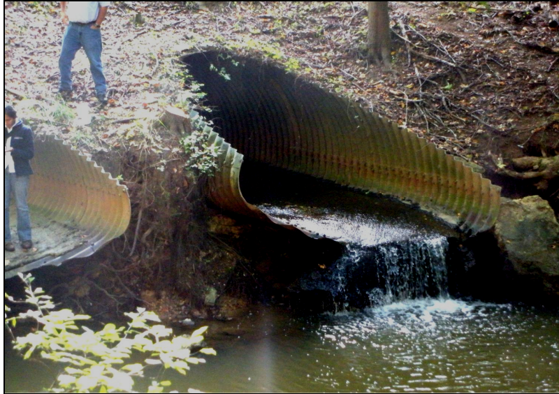
Figure 5.10. Scour at culvert outlet.
