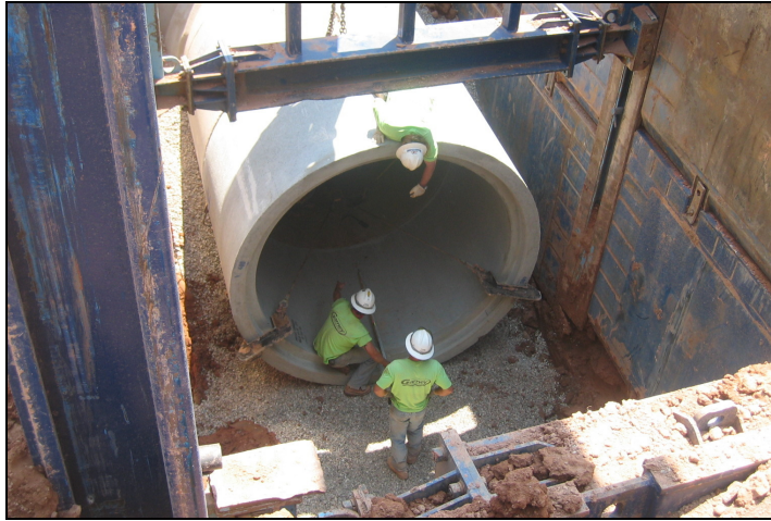
Figure 6.10. Open-trench excavation with shoring.
