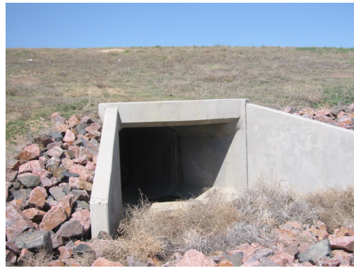
Figure 1.2. Typical concrete box culvert.
