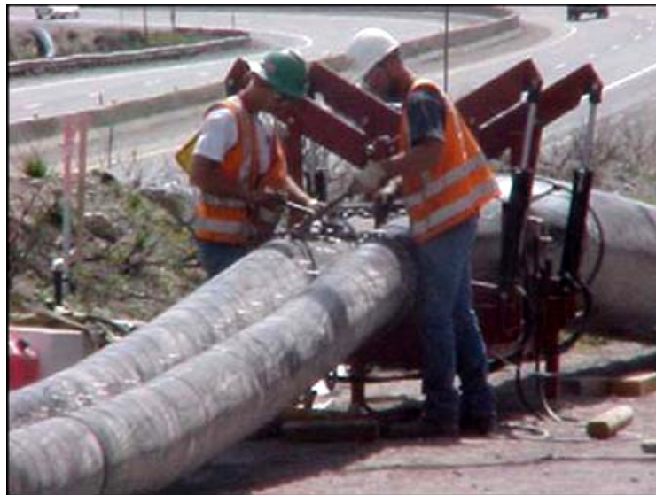
Figure 6.15. Deformed-reformed liner installation.
