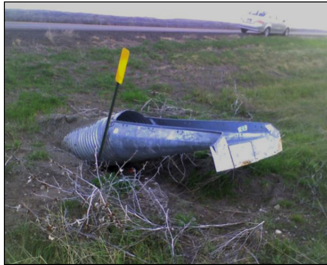
Figure 6.5. Buoyancy uplift.
