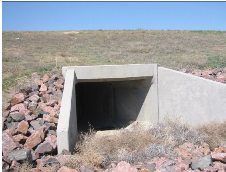
Figure 5.9. Inlet protection based on headwall, wingwalls and riprap.
