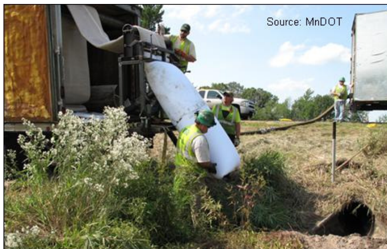
Figure 6.14. Cured-in-place liner installation.
