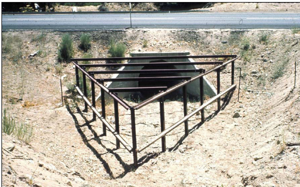
Figure 2.6. Steel rail debris deflector (looking downstream).
