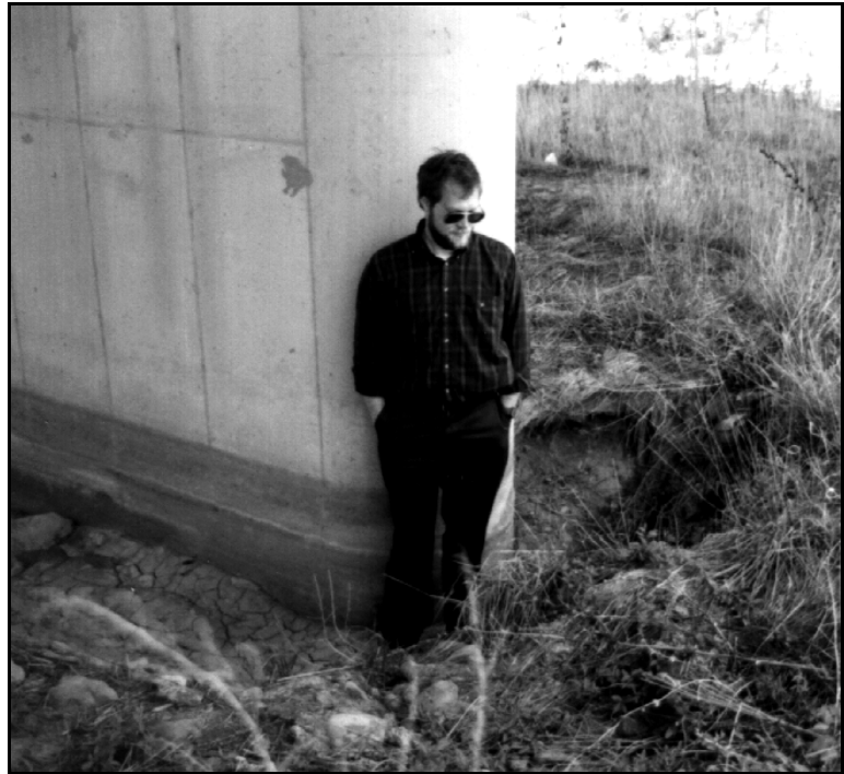
Figure 4-3. Local scour at a round-nosed bridge pier. Note protective vegetative cover of surrounding floodplain.
