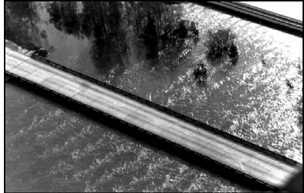
Figure 1-1. A highway bridge that creates complex hydraulic conditions by constricting floodplain flows at high stages.
