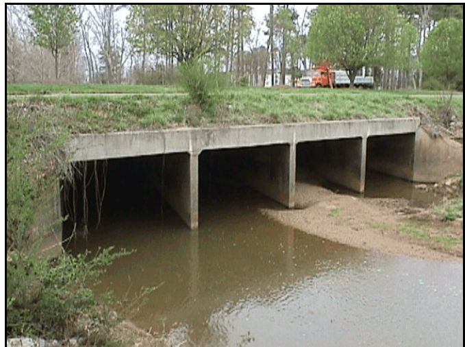
Figure 3-7. Bridges and culverts can be modeled well by one-dimensional flow approximations when their widths are small in comparison to the channel and floodplain.
